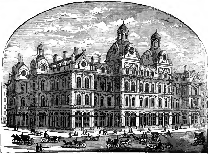
CUSTOM HOUSE AND POST-OFFICE.
