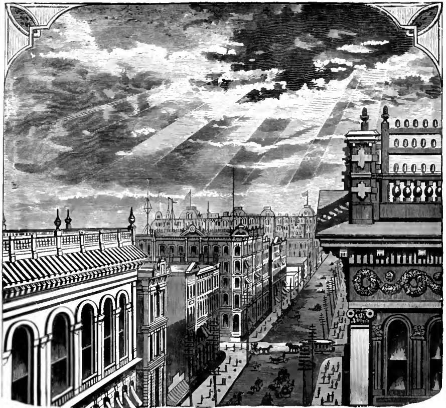
VIEW OF LASALLE STREET, LOOKING SOUTH.
